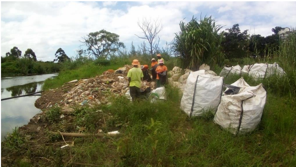
The enormous amount of waste collected since the boom was installed.
